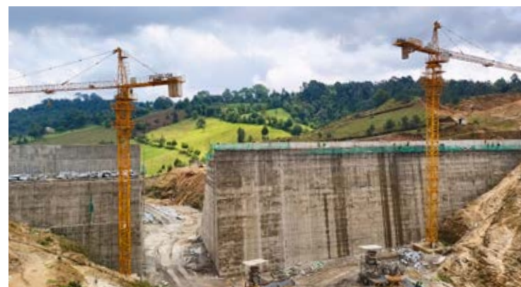
1. Resident Engineer Tabitha Kimani (left) explains the progress of the Muruny (Siyoi) Dam project to Water, Sanitation and Irrigation Cabinet Secretary Eng. Eric Mugaa and other officials using project charts during
